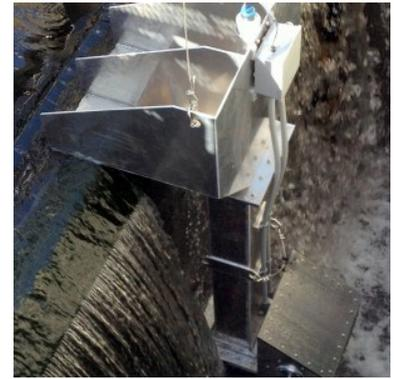
**A Hydrovolts generator installed at West Sound Utility District at Port Orchard. Photo courtesy of the company.**
